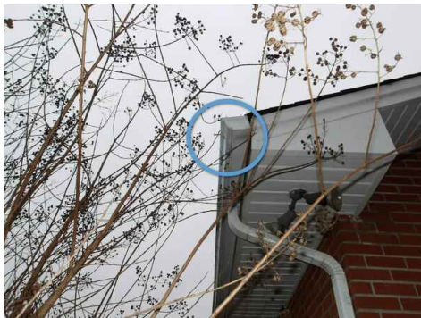
gutter nails coming loose, right front corner
