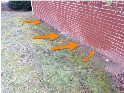
negative soil grade, water not absorbed by the soil will drain toward the foundation, back left of home
