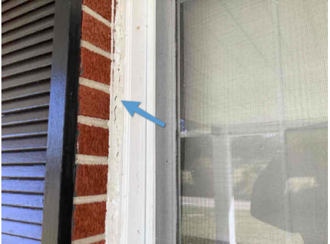
Cracked caulking, side of front living area window
