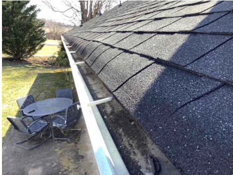
No gutter screening
