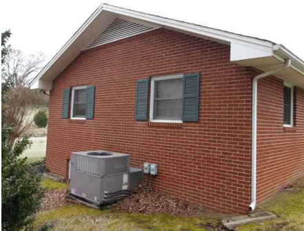
exterior heat pump, right side of home, split system
