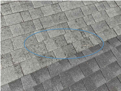
Granules missing, front
