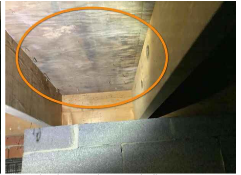
microbial growth on sub floor
