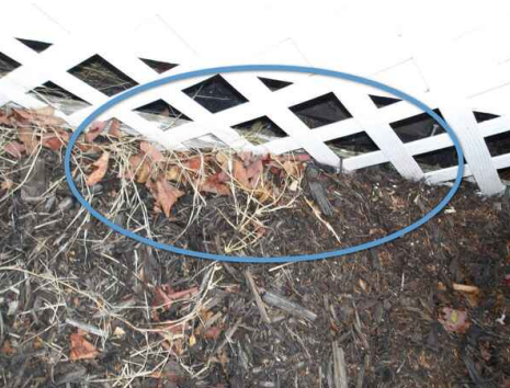
wood framing for front porch skirting framing in soil contact
