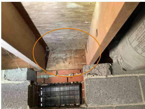
microbial growth on subfloor
