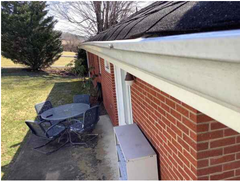
Aluminum gutttering
