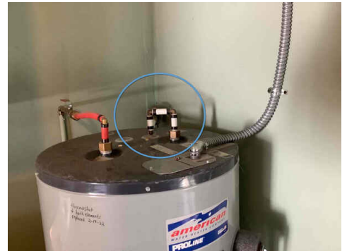
No expansion tank on cold water line
