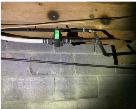
Pressure reducer valve, left side wall of crawlspace
