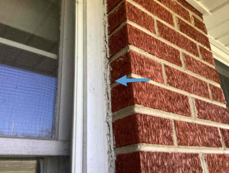
Cracked caulking around some windows, between windows and exterior brick
