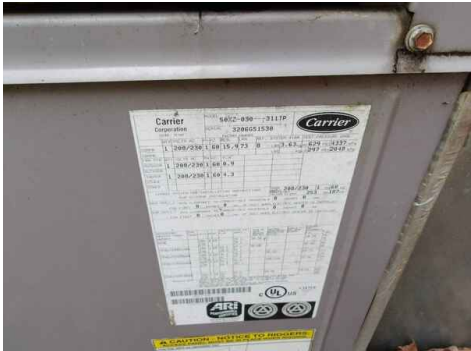
package unit data plate
