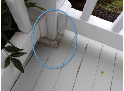
chipped / peeling wood trim at base of front porch railing / covering support post
