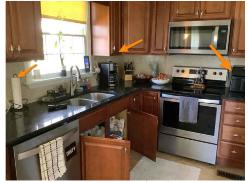
No GFCI protection on kitchen countertop receptacles
