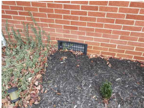
front foundation vent
