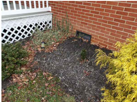
thick layer of mulch, soil grade is not visible, right of front porch
