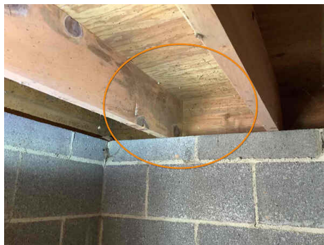
microbial growth on subfloor
