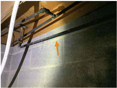
1/2 copper supply lines in crawlspace
