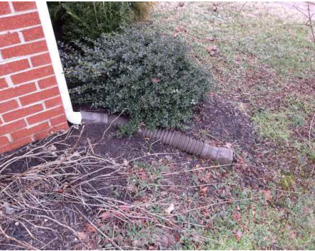
left front corner downspout to surface drain line
