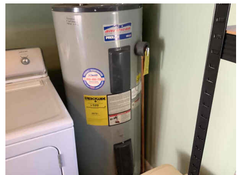
No water heater strapping
