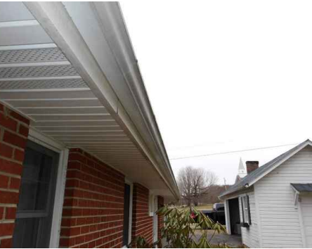
aluminum gutter around the fascia boards
