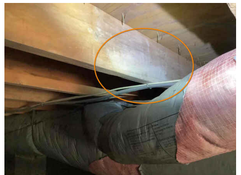
microbial growth on floor joists
