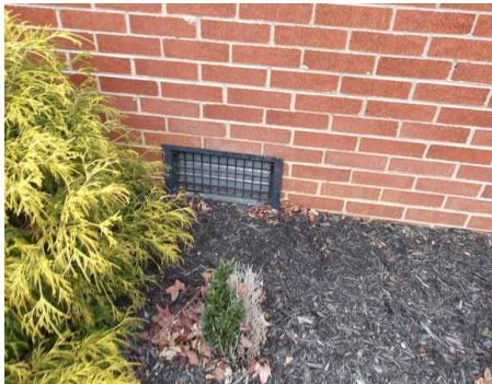
front foundation vent
