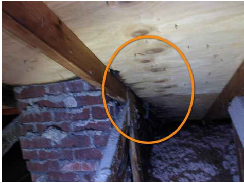
water staining on roof decking around chimney
