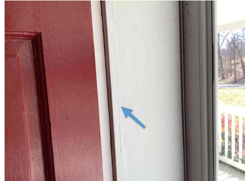
Front entry, hinge side of door casing, no front door casing weather stripping
