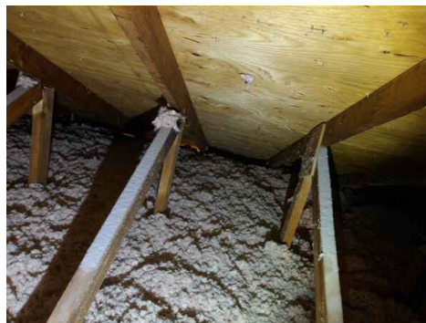
fiberglass loose fill insulation
