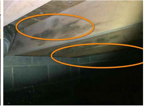
microbial growth on floor joists
