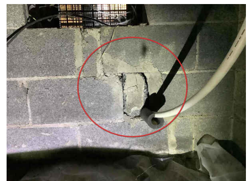
Slight damage with displacement at water line entry, left front foundation
