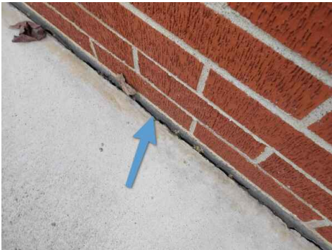
open areas in the space between the back concrete patio and the brick and mortar cladding
