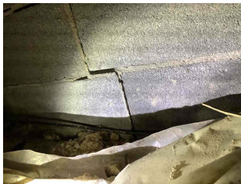
Displacement of the block at the soil line and about 4 blocks up
