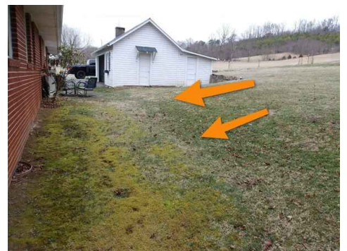
back yard soil grade is negatively sloped toward the home
