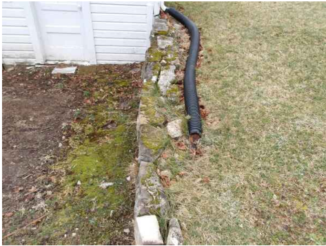
garage gutter downspout releasing water on back side of retaining wall
