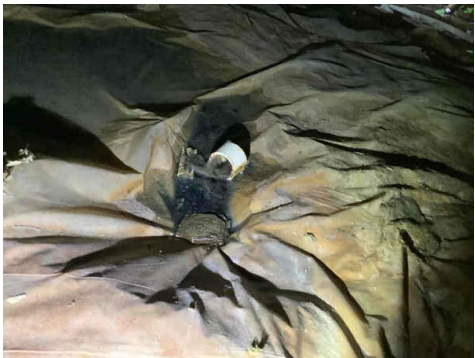
Water on vapor retarder under plumbing leak
