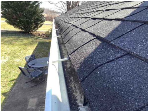
Shingle over hang 2 inches plus, back side
