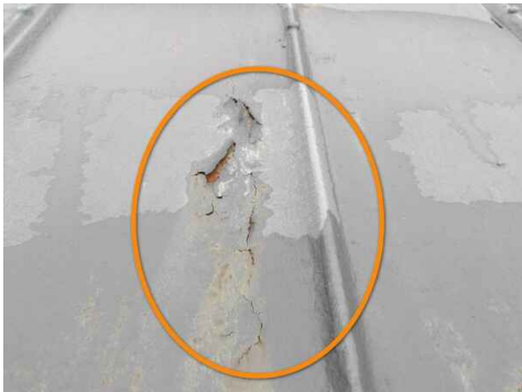
rust / chipped-peeling paint
