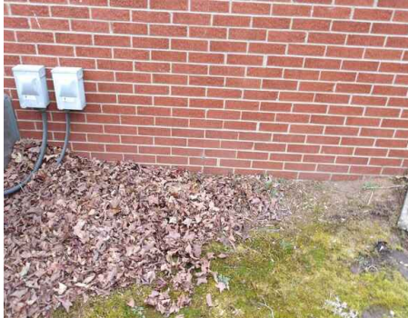
no right side foundation venting
