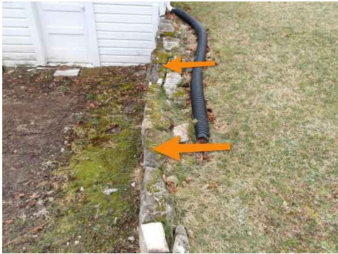
retaining wall slightly leaning, presumably due to soil pressure or hydrostatic (water) pressure
