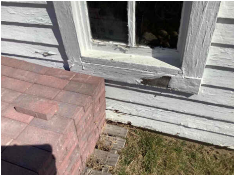
detached garage exterior wood siding, chipped / peeling paint
