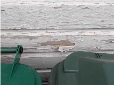
detached garage exterior wood siding, chipped / peeling paint
