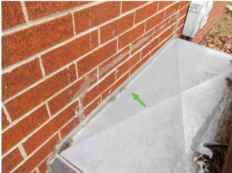
heat pump package unit casing secured to exterior brick cladding
