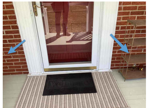
No exterior electrical receptacle, front of home
