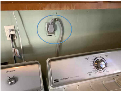
Three pronged versus four pronged dry plug / receptacle
