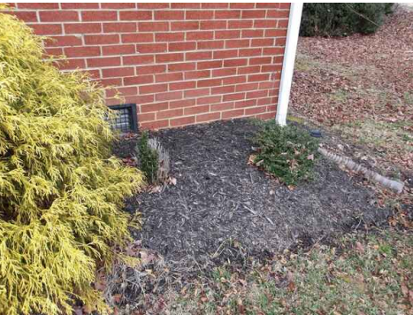
thick layer of mulch, soil grade is not visible, right front of home
