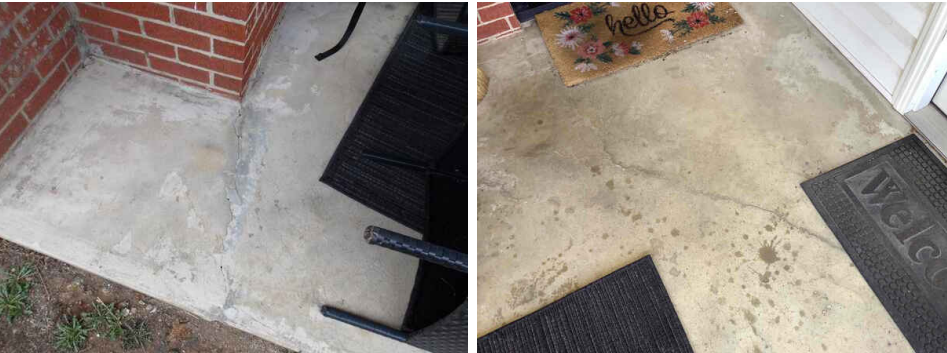
Left side entry concrete slab cracking
