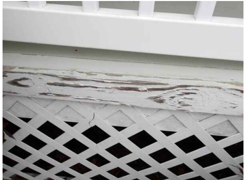
chipped / peeling paint on porch band board
