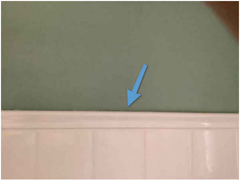
No caulking above shared bathroom shower enclosure
