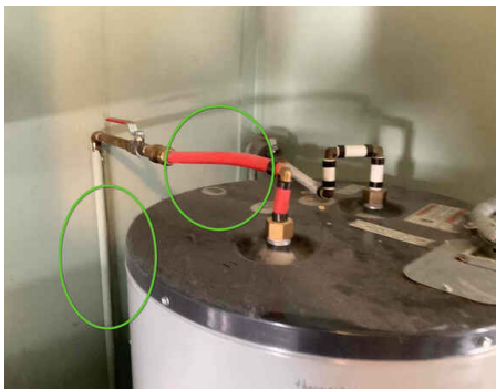
Both Copper and PEX lines
