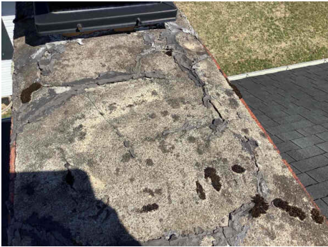
Cracking of chimney crown, cracking of tar used to seal cracks in chimney crown
