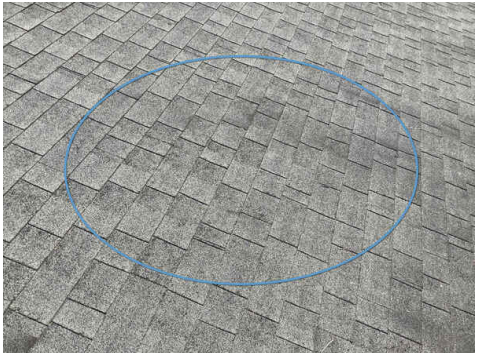
Granule wear, front roof line
