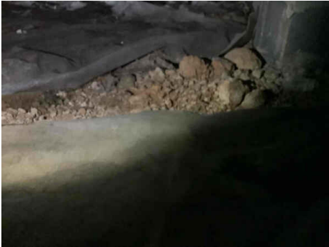
Exposed soil, gaps in plastic vapor retarder
