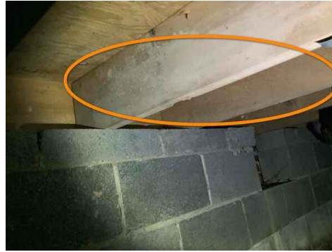
microbial growth on floor joists
