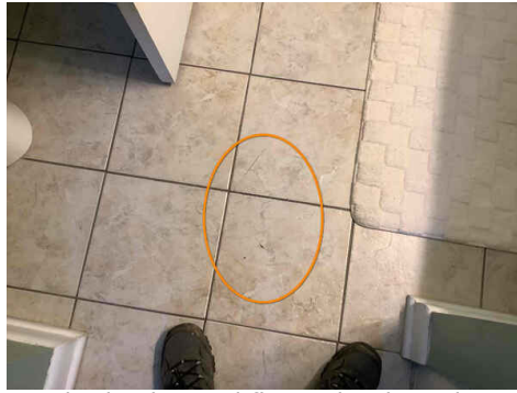
Cracked / chipped floor tile, shared bathroom
