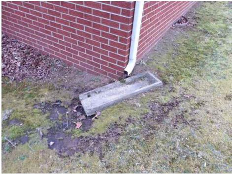
back right downspout to surface drain
