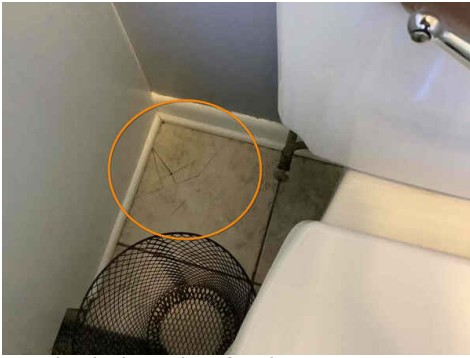
Cracked tile, side of toilet
