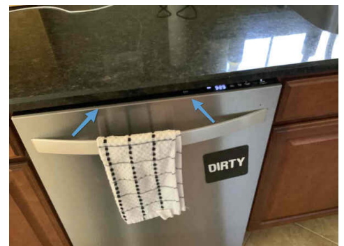
Dishwasher not secured to the underside of the countertop
