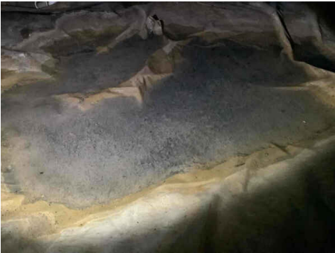
Water puddle under drain lines under back bathrooms
