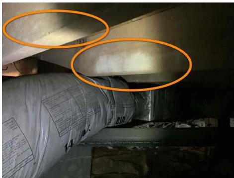
microbial growth on floor joists
