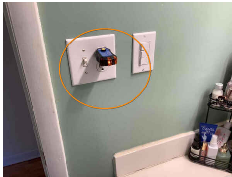
No GFCI protection, hallway shared bathroom
