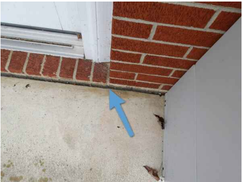
gaps in caulking between back side patio and exterior brick cladding
