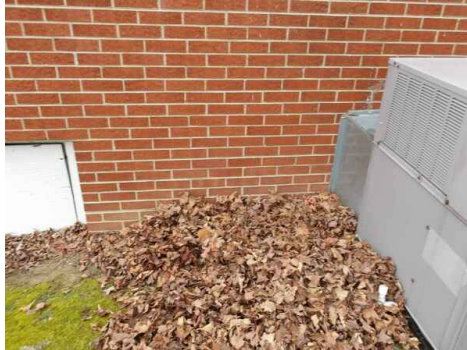
no right side foundation venting
