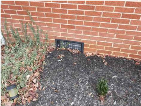
soil / mulch over base of foundation vent, front of home
