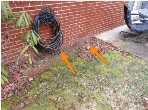
flat soil grade along foundation, back side of the house, left of the back patio
