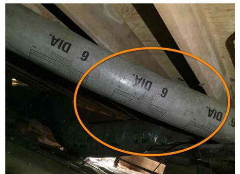
microbial growth on HVAC duct work lines
