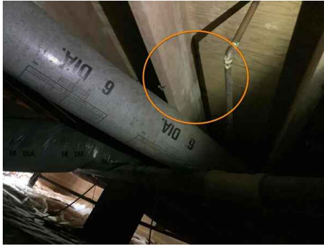
microbial growth on floor joist
