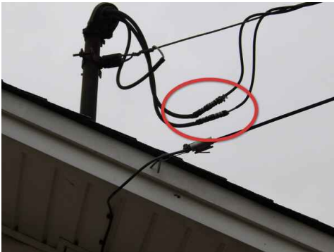
insulation missing on service splices
