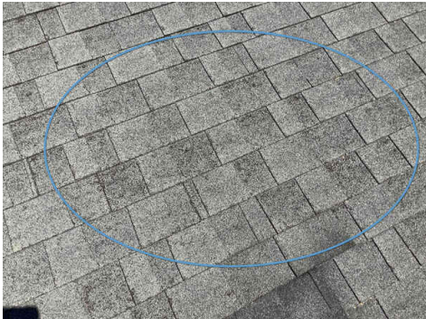
Granule wear, front roof line
