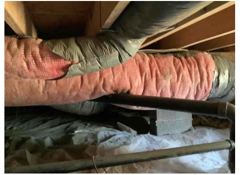
Plastic that secures the duct work insulation is deteriorating
