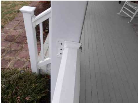
top railing to the right of the front step's connection point is broken
