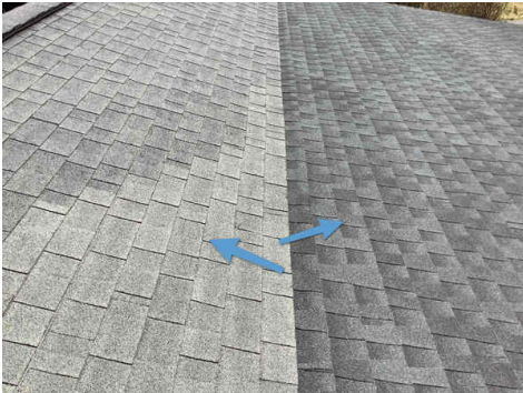
Front porch shingles appear near than the rest of the roof line
