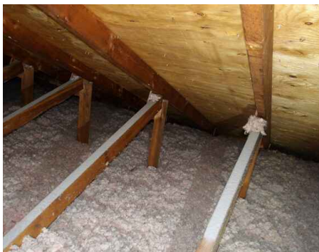
fiberglass loose fill insulation
