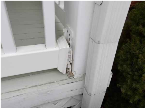
right front corner bottom railing support connection is broken
