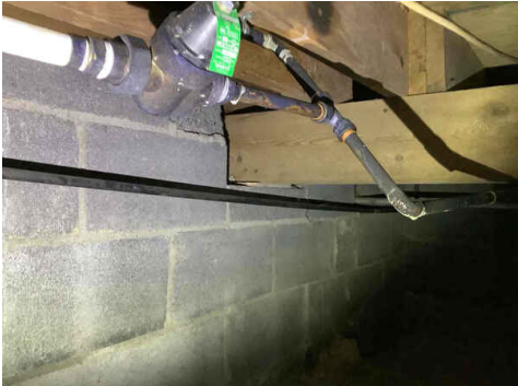
No main water line shut off
