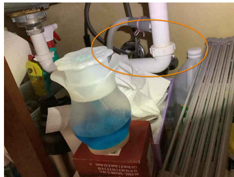
No high loop in dishwasher drain line
