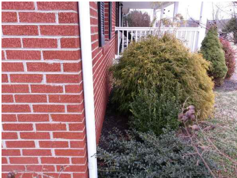
thick layer of mulch, soil grade is not visible, left front of home
