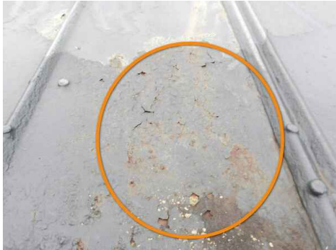
rust, chipped / peeling paint
