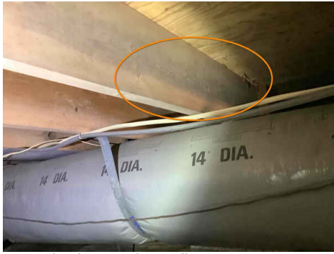
microbial growth on floor joist
