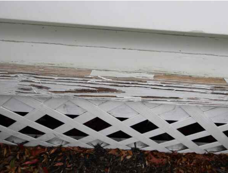
chipped / peeling paint on porch band board
