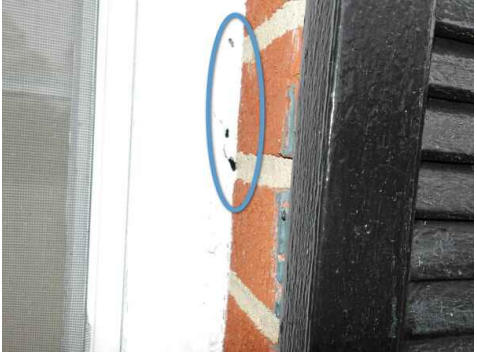
cracks in window / cladding caulking
