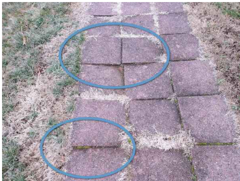
dropped / raised pavers with raised edges
