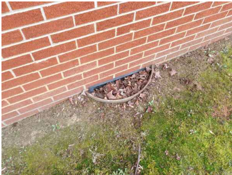
vent well blocked with leaf debris, back left of home
