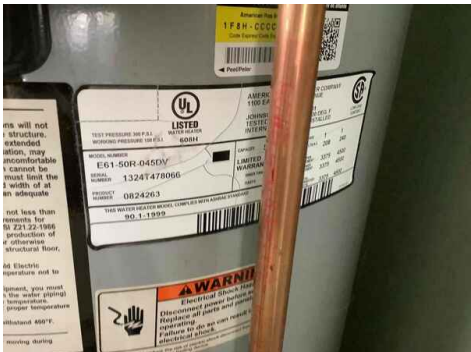
Water heater data plate
