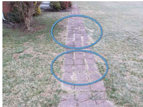
low areas where water may pool, raised and dropped pavers
