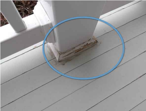
chipped / peeling paint on wood trim at base of porch railing support posts
