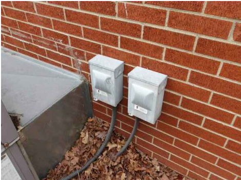
package unit electrical disconnects
