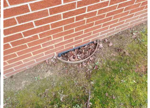
back right foundation vent, only vent on the back crawlspace foundation
