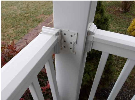
left front top railing connection point broken
