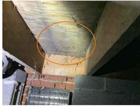
microbial growth on sub floor
