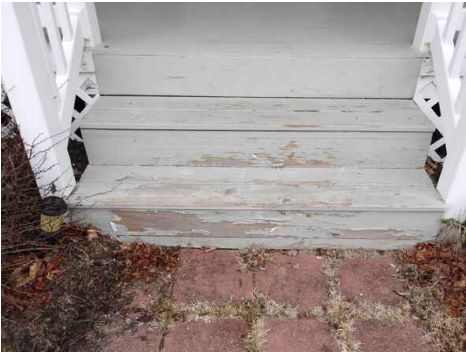
chipped / peeling paint on front porch stairs
