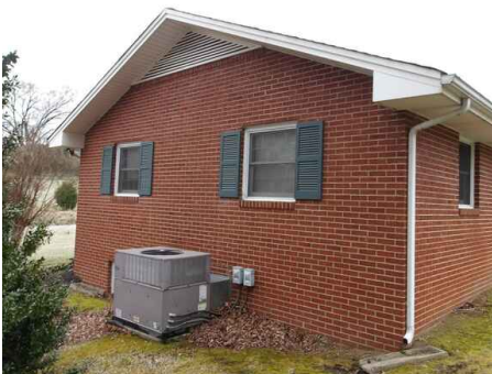
heat pump package unit, right side of house
