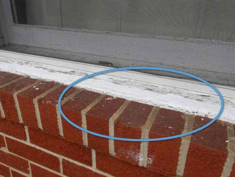
cracking in existing window caulking
