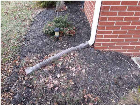
right front corner downspout to surface drain line
