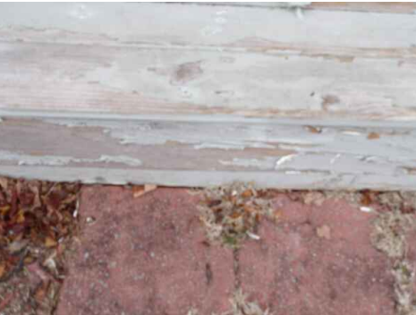
chipped / peeling paint on front porch stairs
