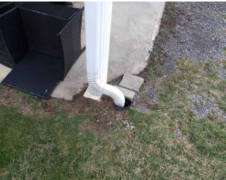
back left downspout to sub drain line
