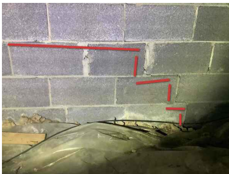
Vertical and stair step cracking, front foundation wall, left of front door, displacement of the block around the cracking
