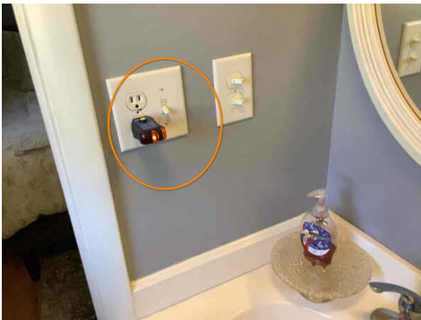
Primary bathroom, vanity receptacle, no GFCI protection
