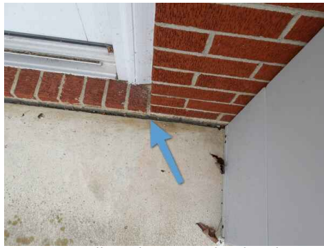
gaps in caulking between back side patio and exterior brick cladding
