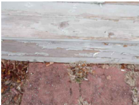
chipped / peeling paint on front porch stairs
