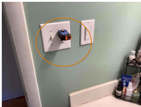
No GFCI protection, hallway shared bathroom
