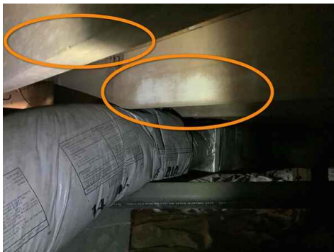
microbial growth on floor joists
