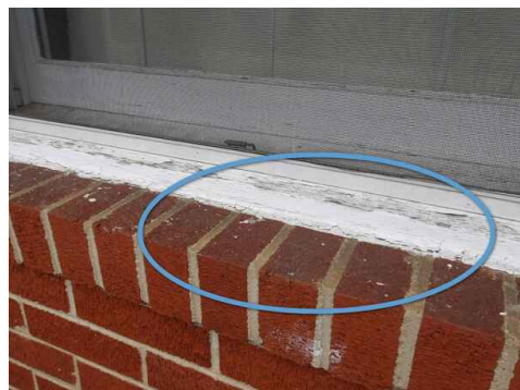
cracking in existing window caulking
