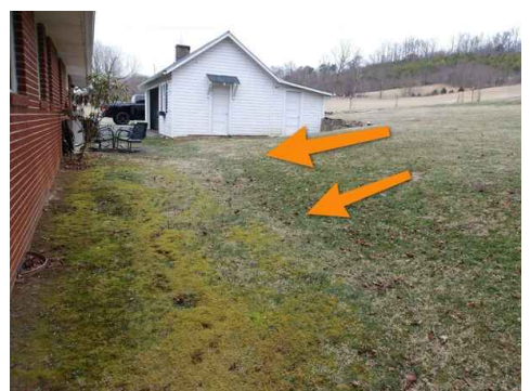
back yard soil grade is negatively sloped toward the home
