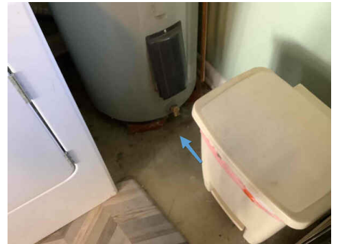
No drip pan under water heater
