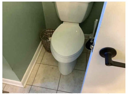
Shared bath toilet, very loose on the floor
