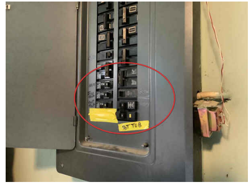
GE and Siemens breakers in an I-T-E panel
