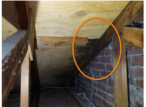
water staining on roof decking on side of chimney
