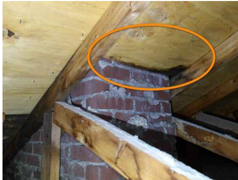
water staining on roof deck at uphill side of chimney
