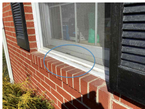
Chipped / peeling paint, front laundry room window
