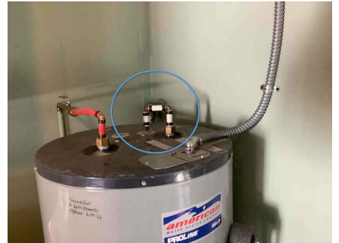
No expansion tank on cold water line
