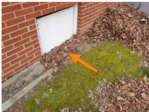
relatively flat soil grade, at base of foundation, right side of home
