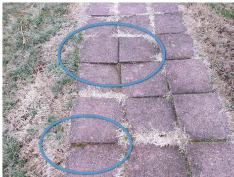
dropped / raised pavers with raised edges
