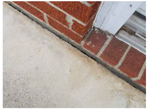
gaps in caulking in gap between patio and exterior brick cladding
