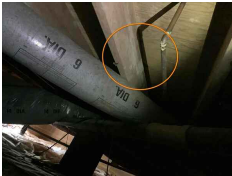
microbial growth on floor joist
