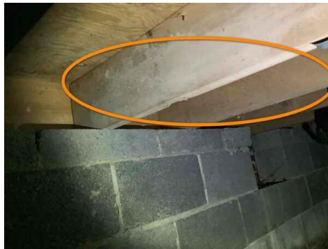
microbial growth on floor joists
