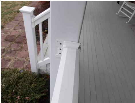
top railing to the right of the front step's connection point is broken
