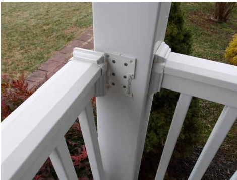
left front top railing connection point broken
