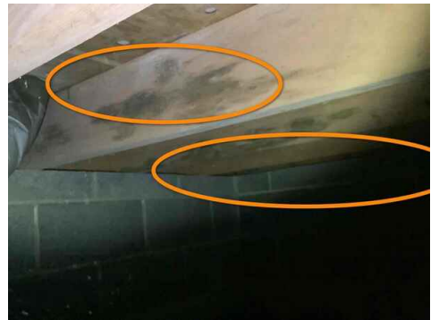
microbial growth on floor joists
