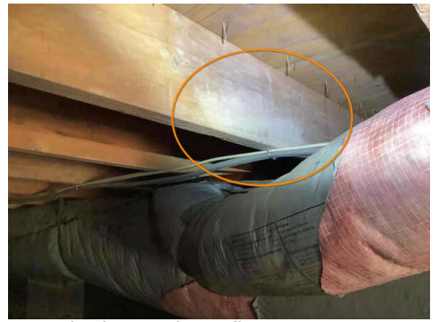
microbial growth on floor joists
