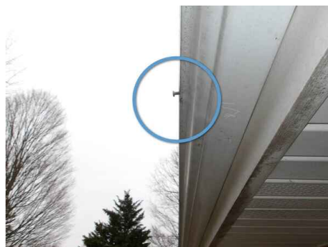
gutter nail coming loose, back left of home
