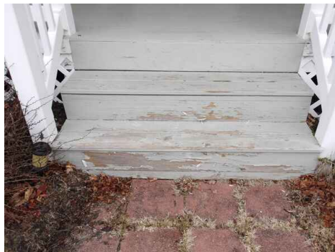
chipped / peeling paint on front porch stairs
