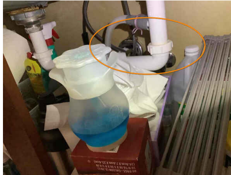
No high loop in dishwasher drain line
