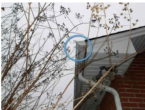
gutter nails coming loose, right front corner
