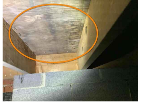
microbial growth on sub floor
