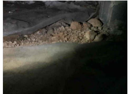
Exposed soil, gaps in plastic vapor retarder
