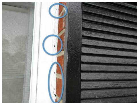
crack / gaps in window caulking
