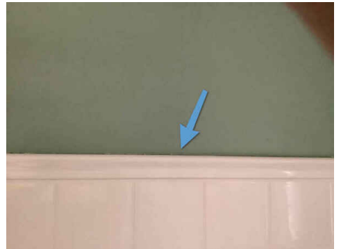
No caulking above shared bathroom shower enclosure
