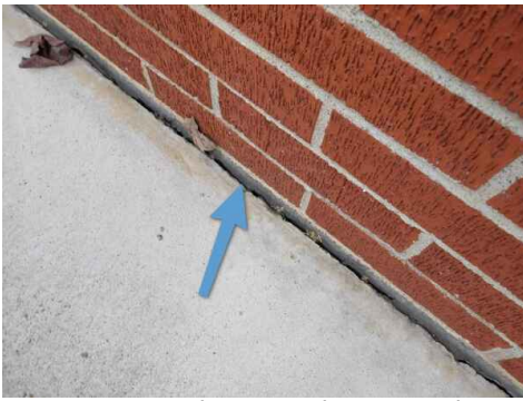
open areas in the space between the back concrete patio and the brick and mortar cladding
