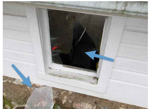
broken window pane, back side of detached garage
