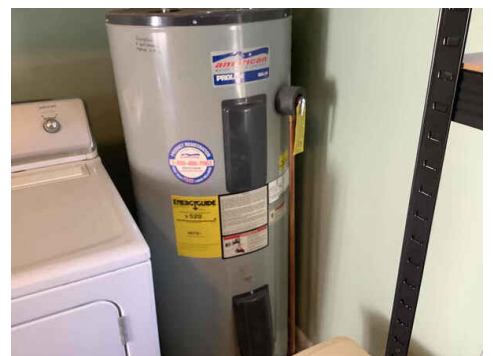
No water heater strapping
