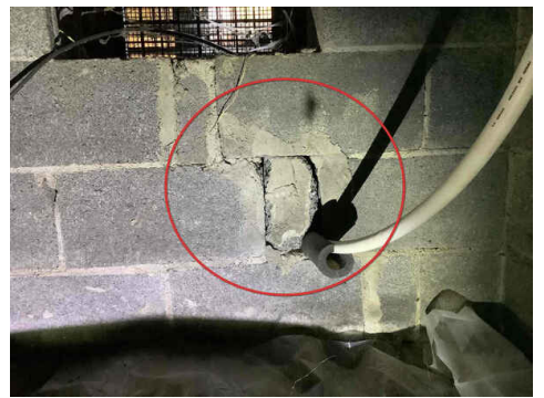
Slight damage with displacement at water line entry, left front foundation
