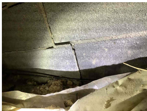
Displacement of the block at the soil line and about 4 blocks up
