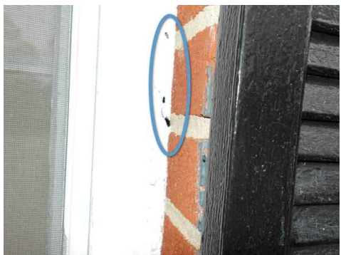
cracks in window / cladding caulking
