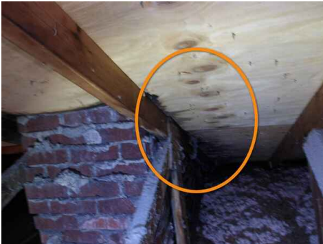
water staining on roof decking around chimney
