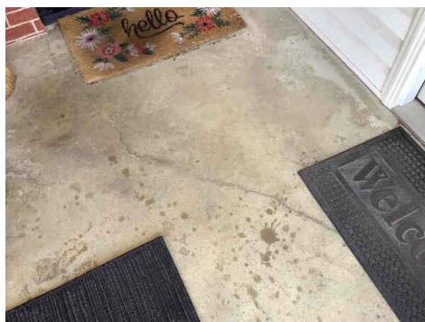
Left side entry concrete slab cracking
