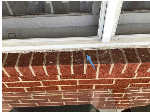
Cracked caulking, base of front living area window
