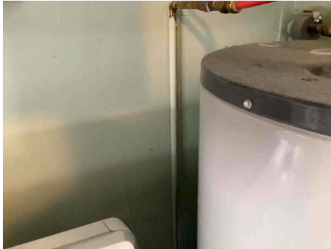
Copper water distribution lines at the water heater are 1/2 inch copper lines, versus 3/4 inch lines
