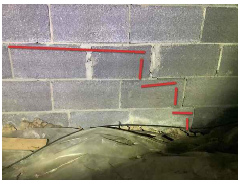
Vertical and stair step cracking, front foundation wall, left of front door, displacement of the block around the cracking
