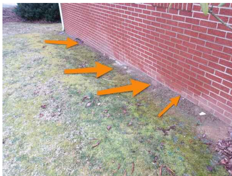
negative soil grade, water not absorbed by the soil will drain toward the foundation, back left of home
