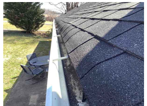
Shingle over hang 2 inches plus, back side
