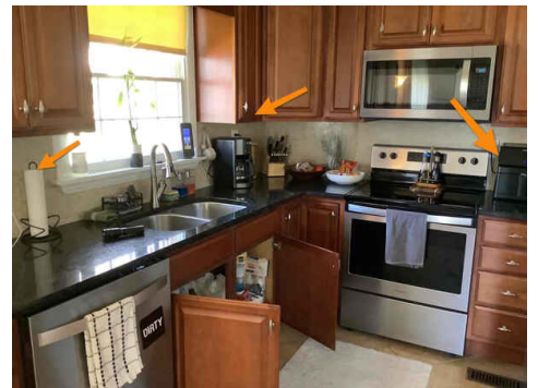
No GFCI protection on kitchen counter top receptacles
