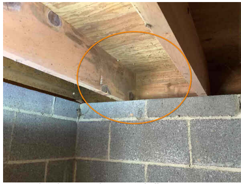
microbial growth on subfloor
