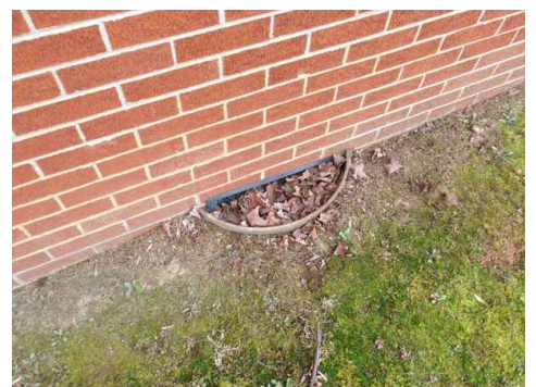
vent well blocked with leaf debris, back left of home
