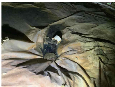
Water on vapor retarder under plumbing leak
