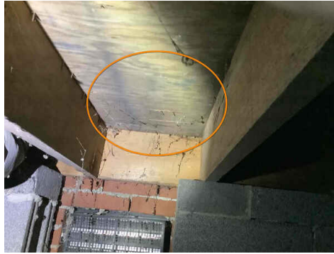
microbial growth on sub floor
