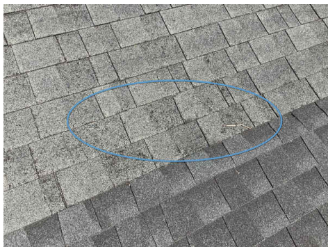
Granules missing, front
