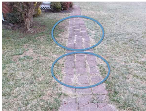
low areas where water may pool, raised and dropped pavers
