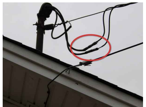
insulation missing on service splices
