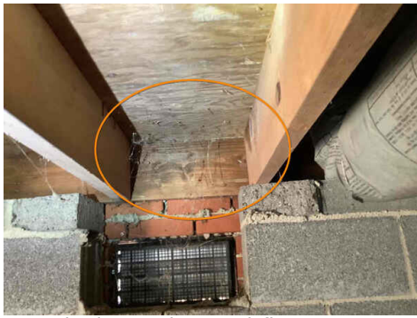
microbial growth on subfloor
