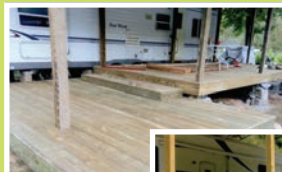
Framing and decking endgrains are covered with band board
