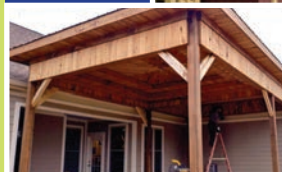
Framing and decking endgrains are covered with band board
