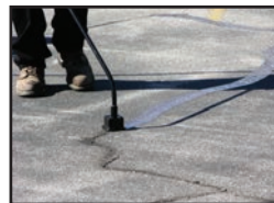
CRACK FILLING
