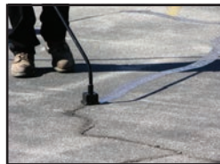
CRACK FILLING
