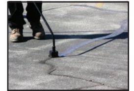
CRACK FILLING
