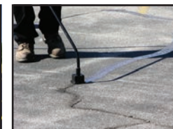
CRACK FILLING
