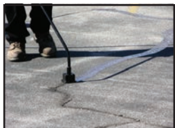
CRACK FILLING
