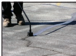
CRACK FILLING
