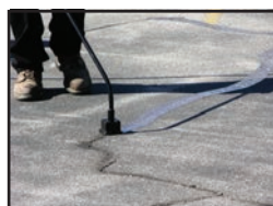
CRACK FILLING
