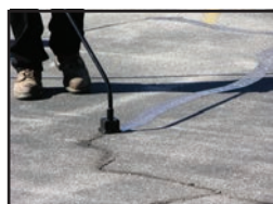
CRACK FILLING
