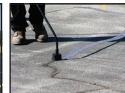
CRACK FILLING
