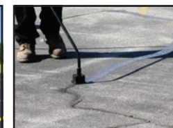
CRACK FILLING
