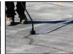
CRACK FILLING
