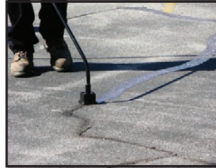
CRACK FILLING
