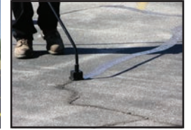
CRACK FILLING
