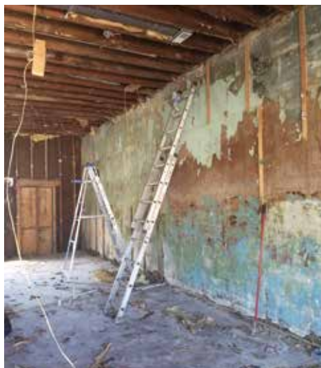
Renovation of the Pioneers building.
