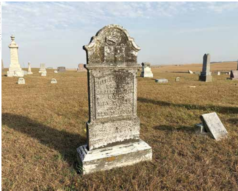
This headstone in Moffitt Grove Cemetery shows how weather can impact the material.
