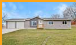
New Construction: 201 NW 3rd Street, Panora
