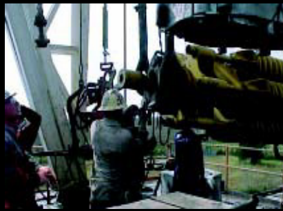
The crew of Patterson Rig 50 rig-up Vibration Technology's 500K oscillator.
