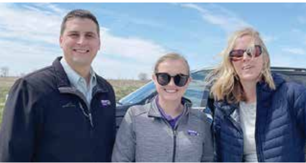
Greg Grote, Ciara Halverson and Jennifer Brown at the groundbreaking for Brilliant Boardsers Landscaping on April 19.
