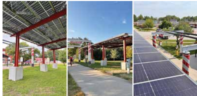
Solar panels provide shade for bicyclists and power for nearby city facilities including the stage in the park.
