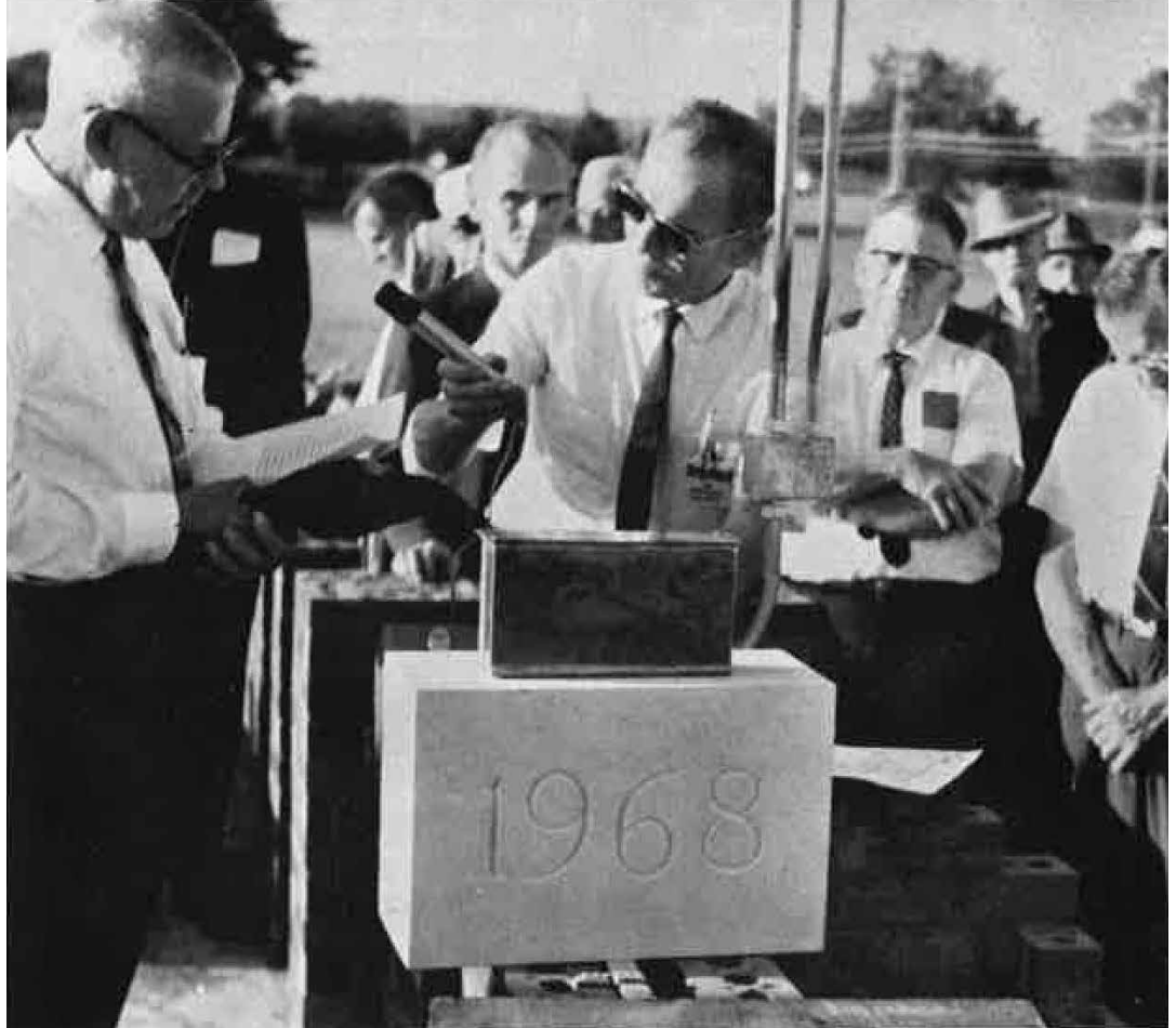
Men's Garden Clubs of America chose 5560 Merle Hay Road in Johnston as the site for the group's national headquarters. Groundbreaking and completion of that headquarters took place in 1968. The cornerstone-laying ceremony took place in 1968. Dr. John B. Miller, President of the Men's Garden Club of Des Moines, speaks, while Herb Plambeck, with the help of his WHO microphone, assists with the ceremony.
