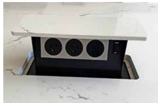
Neal Logan installed a popup outlet on the kitchen island.
