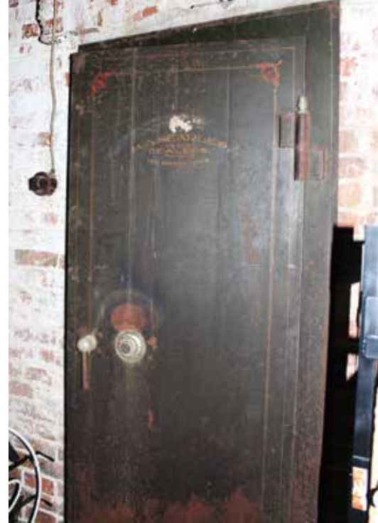
The building now home to Norm’s Pub was once a bank, and the vault is still in the basement. Photo by Jackie Wilson
