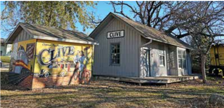
The historic depot was moved a short distance from its original 1882 location after the Clive Historical Society gained possession from the Norfolk Southern Railroad.
