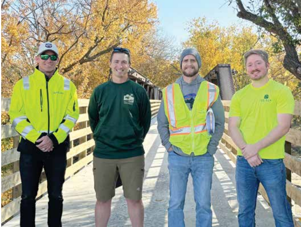
Mike Vaniten (project manager), Tyler Jensen, Curt Cable and Dylan Graber completed the wooden railings on the RRVT lighted bridge at Adel. Photo by Rachel Harrington
