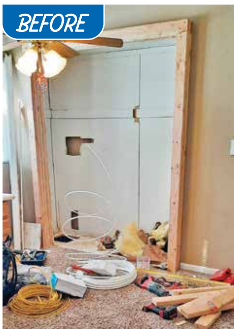
Marilyn Merrell needed a main-level laundry space, so she converted a closet for that purpose. The closet was made deep enough by building out the frame to accommodate the washer and dryer.
