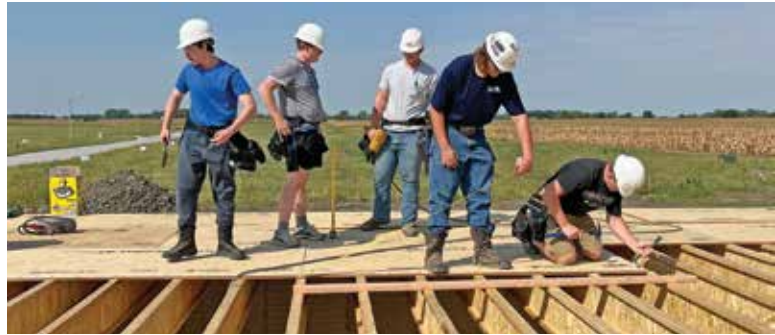
Students in the Construction Technology program build a house.
