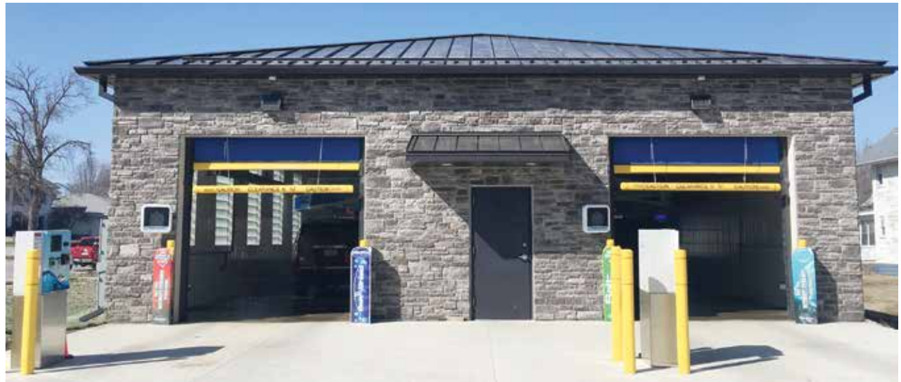
Entrances to the two automatic bays are on the south side of the building. A stone exterior and windows in the west bay make the building more appealing.
