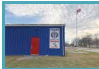
Stuart American Legion, Post 146 New heating and cooling system
