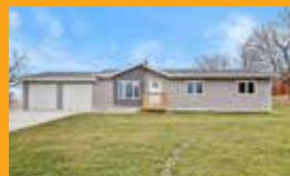
New Construction: 201 NW 3rd Street, Panora
