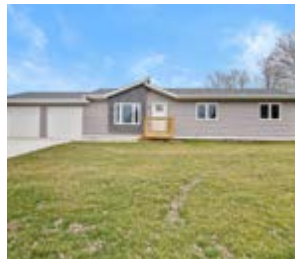
New Construction: 201 NW 3rd St, Panora
