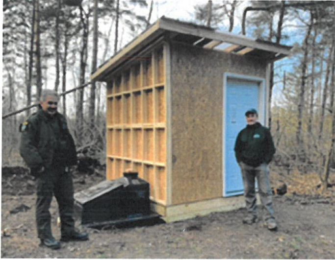
Photo 3: a new restroom near Stirnie Rd
