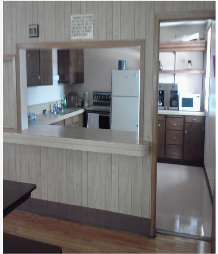
MEMORIAL HALL UPSTAIRS KITCHEN
