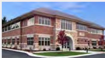
This example shows an office building with a primary facade using brick with stone as an accent material, meeting desired natural color palette.
