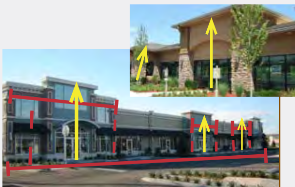
The images above illustrate techniques used to vary the facade heights along a long facade.
