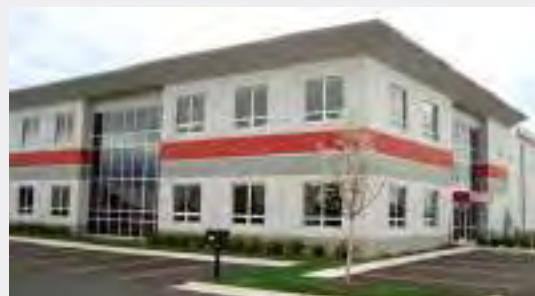
An example of a high quality office building using variations in building color, projections and windows to break up long walls.
