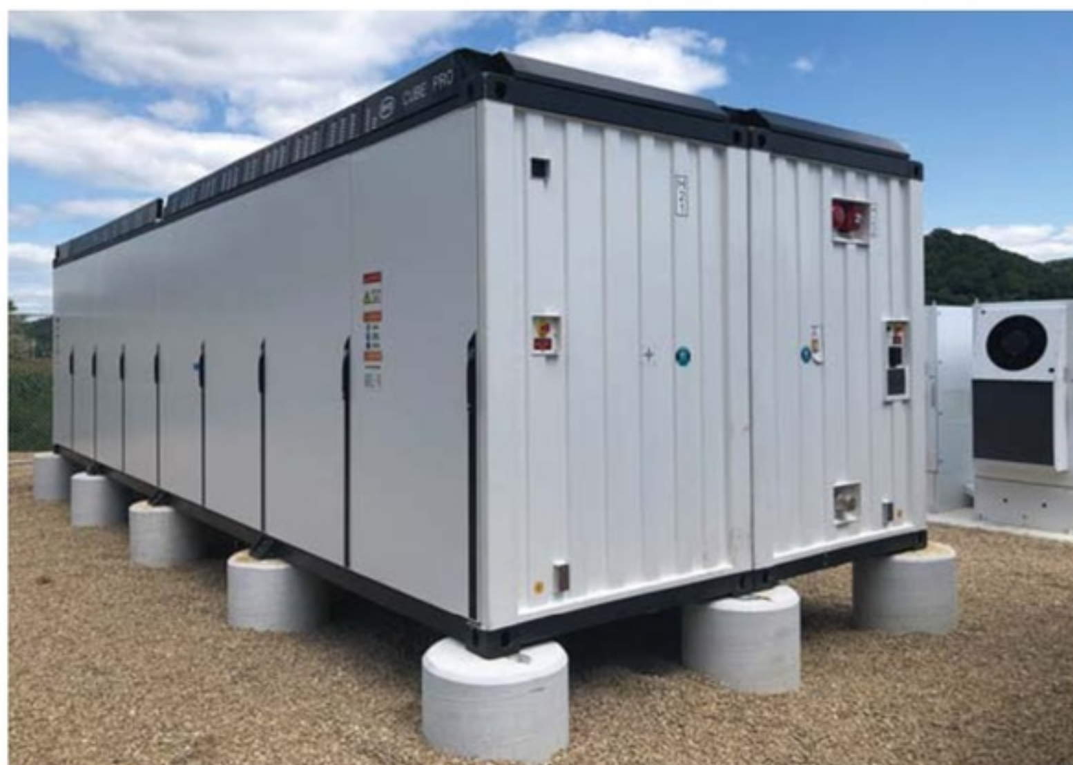
The microgrid relies on two 1.6-MWh lithium-iron-phosphate battery (LFP) modules, for a combined 3.2 MWh of energy storage capacity.
