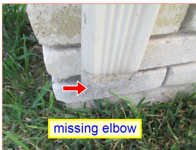
B. Item 8(Picture) Front of Home
