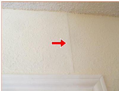
E. Item 10(Picture) hallway - example photo
