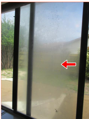
H. Item 9(Picture) Bedrooms (sleeping areas) North Side
