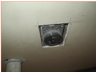
B. Item 8(Picture) laundry room
