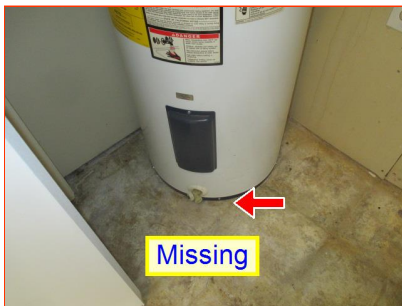
C. Item 1(Picture) laundry room
