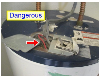
C. Item 2(Picture) laundry room
