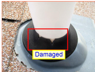
C. Item 2(Picture) rooftop
