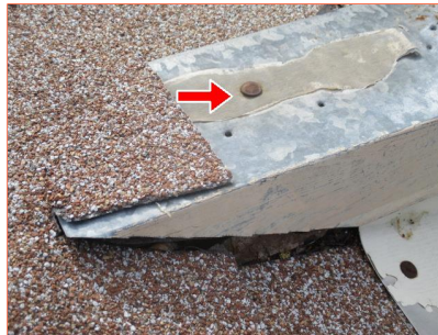
C. Item 5(Picture) rooftop
