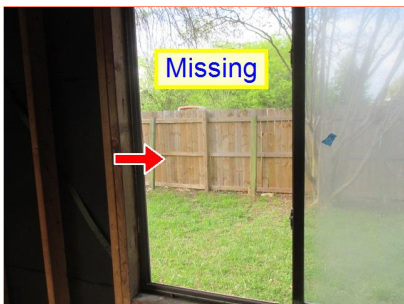
H. Item 2(Picture) Rear of Home
