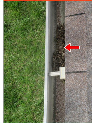
B. Item 12(Picture) Rear of Home
