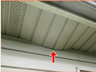
D. Item 1(Picture) Rear of Home
