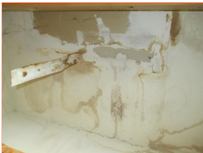
F. Item 1(Picture) garage
