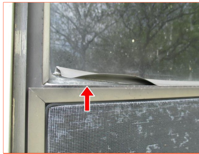
H. Item 8(Picture) Rear of Home
