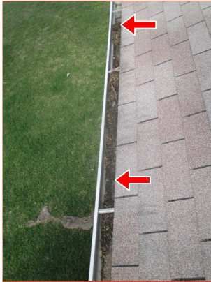
B. Item 10(Picture) right side (facing front) Front of Home
