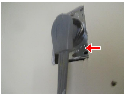
B. Item 9(Picture) laundry room
