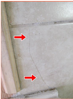
F. Item 10(Picture) Kitchen
