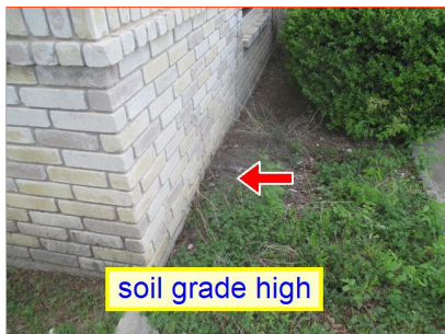
B. Item 1(Picture) Front of Home
