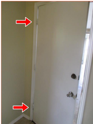
G. Item 3(Picture) garage small door
