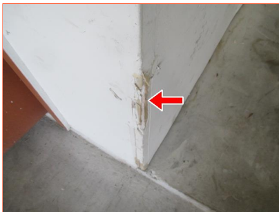
E. Item 9(Picture) garage
