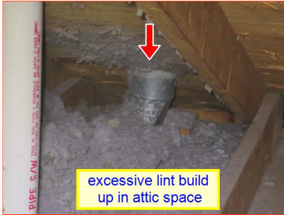
H. Item 1(Picture) attic space
