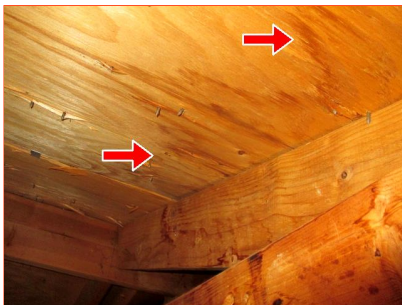
D. Item 3(Picture) attic space
