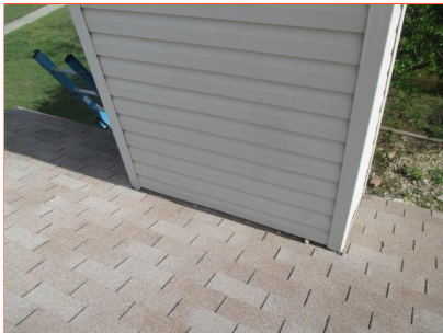
J. Item 1(Picture) rooftop
