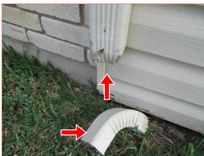
B. Item 7(Picture) right side (facing front) Rear of Home
