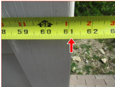
J. Item 2(Picture) chimney chase
