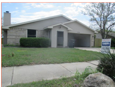
E. Item 3(Picture) water meter location
