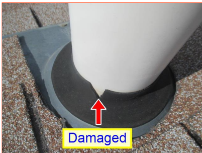
C. Item 1(Picture) rooftop
