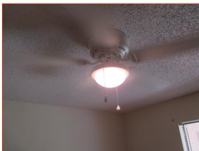
B. Item 20(Picture) Rear of Home bedroom
