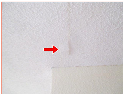
F. Item 5(Picture) Rear of Home
